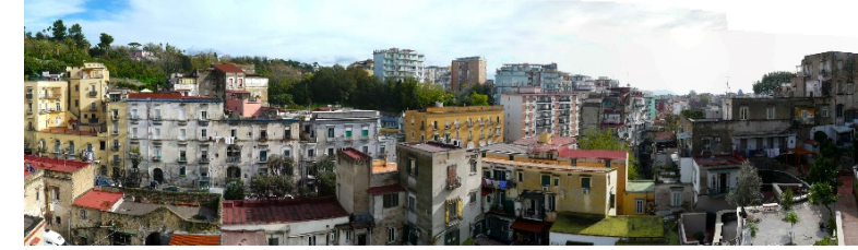
Infrastructure barrier for urban cohesion (social & economic) Corso Amedeo Di Savoia
